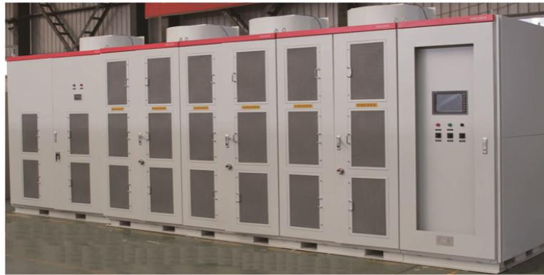
Fig. (9). High voltage STATCOM site.
