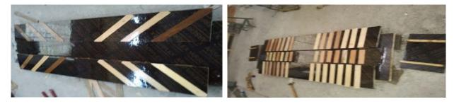
Fig. (4). Preparations of molds for vertical and inclined CFRP for B4 and B5.
