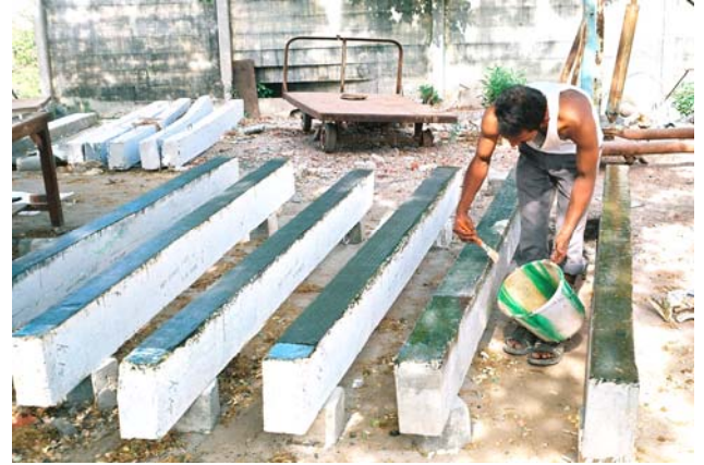
Fig. (3). Finished with Protective Coating Over Second Layer.
