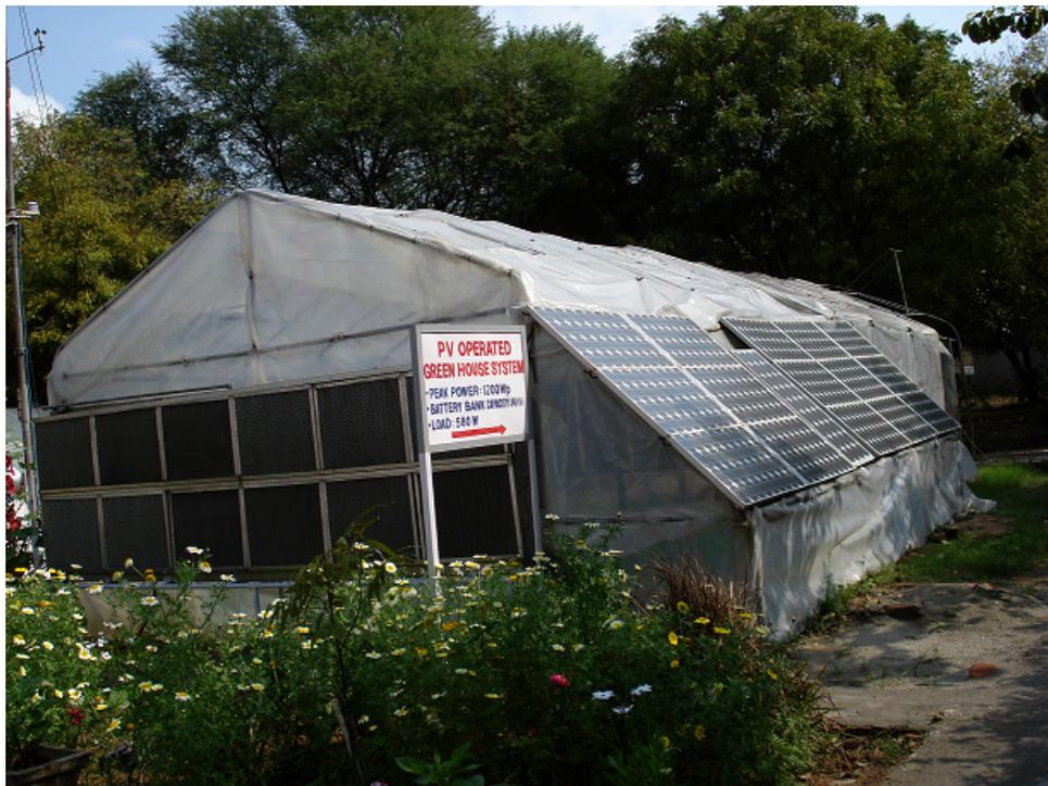
Fig. (3). PV integrated greenhouse system with evaporative cooling.
