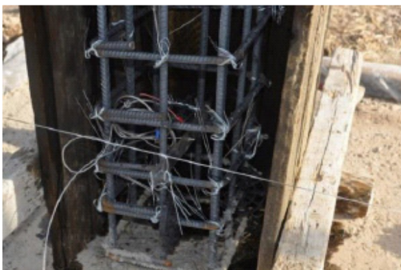
Fig. (3). Insertion of a thermocouple.
