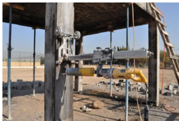
Fig. (6). Core location in reinforced concrete frame.
