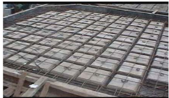
Fig. (1). Reinforced concrete honeycombed-core girderless floor.
