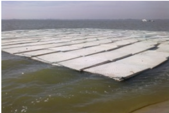
Fig. (3). Motion behavior of the polystyrene board coverage structure under level-6 wind wave.
