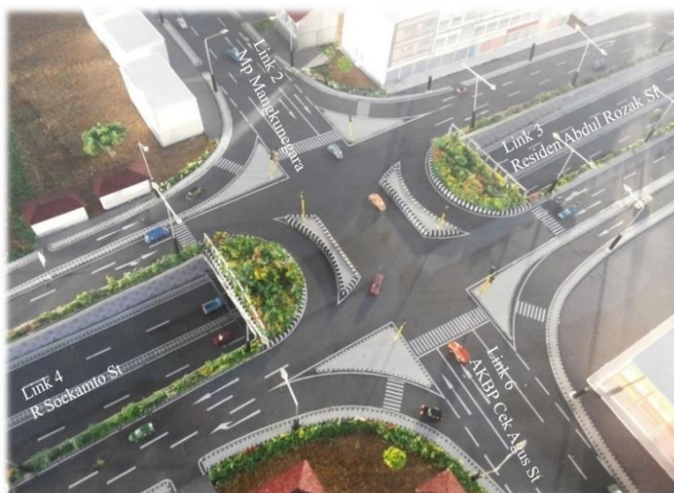
Fig. (2). Underpass construction at Patal-Pusri intersection.
